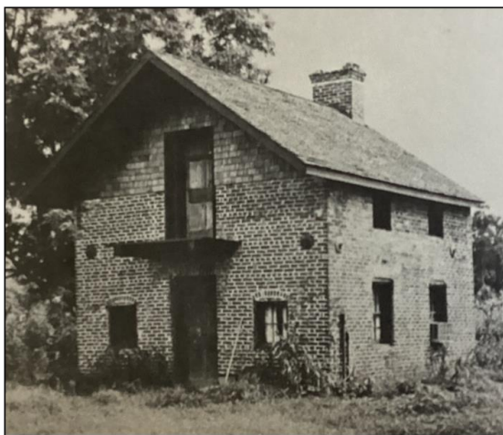
Pavilions erected for accommodations of guests, ca. 1760 Courtesy Historic Preservation Inventory, Berkeley County, 1979
