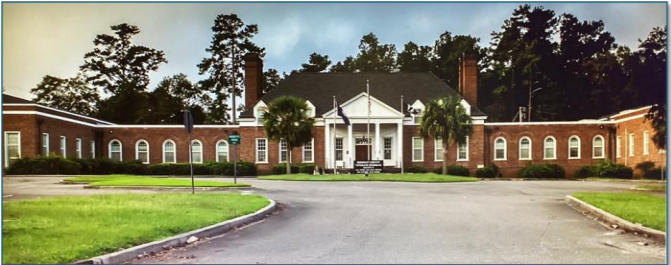
Old Berkeley County Hospital 2019, courtesy Brandon Coffey
