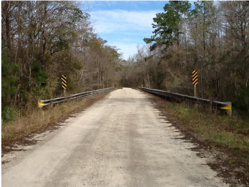
Wambaw Creek Bridge (today)
